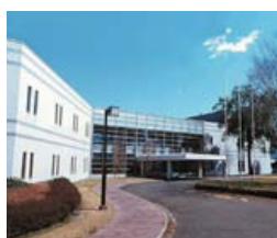
Nippon Meat Packers' Research & Development Center, located in Tsukuba, the 'science city' in Ibaraki Prefecture.
