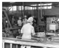
Plant interior at the time
