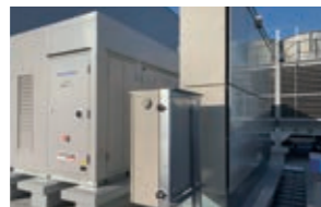
Fluorocarbon-free refrigeration units at Nippon Daily Net Co., Ltd.'s Nagoya 2nd Center
