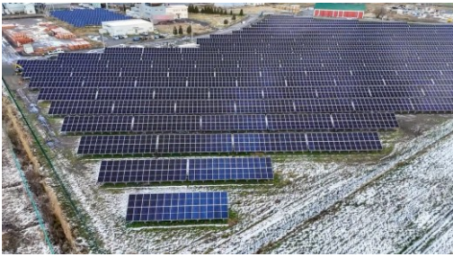
Installation of solar panels
