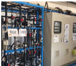
Wastewater recycling using RO membrane processing
