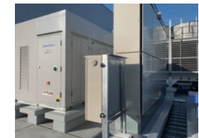
Nippon Daily Net Co., Ltd.'s Nagoya 2nd Center Fluorocarbon-free refrigeration units
