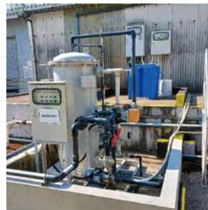
Rainwater filtration equipment
