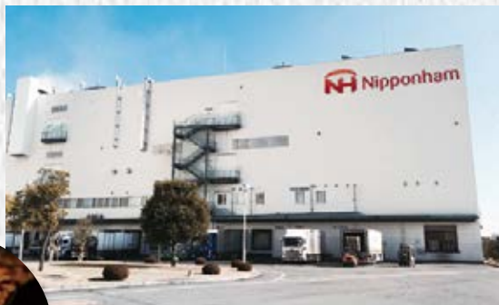
Ibaraki Plant, Nipponham Factory Ltd.
