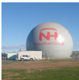
Biogas plant of Oakey Beef Exports Pty. Ltd.
